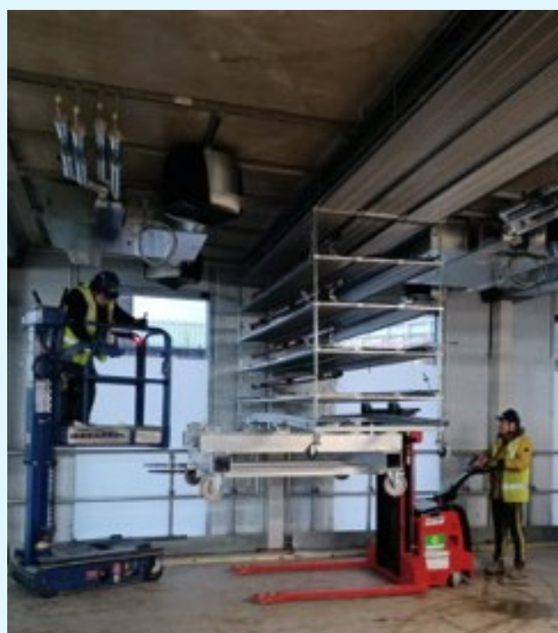
FIGURE 5 – Use of stillages and lifting equipment to improve installation productivity
